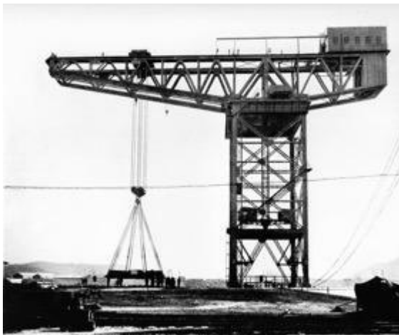
Figures 17 and 18: The completed Sasebo Giant Cantilever Crane undergoing testing after its completion in 1913. Although its official capacity was 250 tons, it was tested up to 312 tons with the help of the shipyard workforce (Images: Brian Newman)
