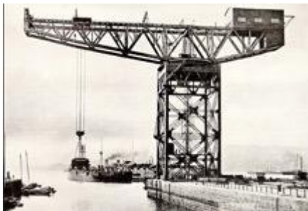
Figures 9, 10 and 11: Giant Cantilever Cranes at Kure (1911), Yokosuka (1911), and Yokohama (1913), all built by Cowans Sheldon of Carlisle, England (Images: Brian Newman and Miles Oglethorpe)
