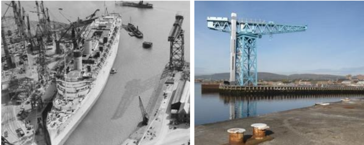
Figures 14 and 15: the 150-ton Giant Cantilever Crane built at John Brown’s Shipyard in 1908 by Sir William Arrol. The view on the left shows the Queen Mary ocean liner being fitted out. Today, the crane is all that survives of the historic shipyard. (Images ©Courtesy of HES)
