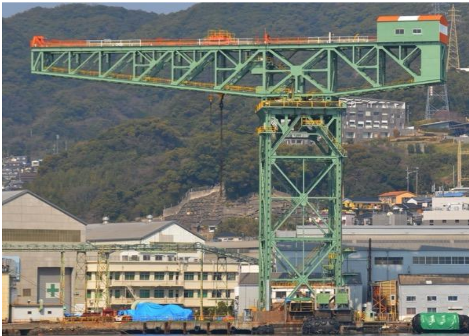
Figure 6: The 150-ton Giant Cantilever Crane at Nagasaki, built in 1909 and still operating within Mitsubishi Heavy Engineering’s shipyard. It was included within the successful UNESCO World Heritage nomination of the Sites of Japan’s Meiji Industrial Revolution in 2015 (Photo: Miles Oglethorpe)
