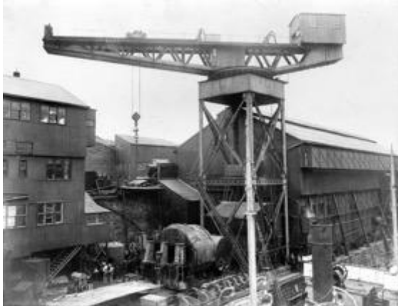
Figures 7 and 8: the first Giant Cantilever Crane was built in 1904 at MacColl & Pollock's shipyard in, Sunderland, England, was 60-ton capacity, and was built and designed by the Glasgow Electric Crane & Hoist Co (Images: Brian Newman)
